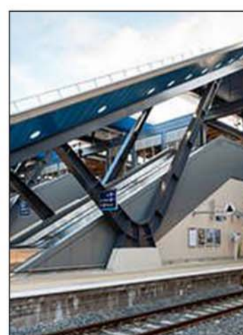
Train station stairwell
