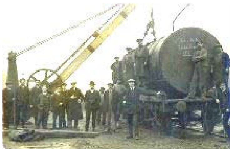
Delivery of the new boiler to the Pelabon Works through Twickenham Goods Yard, December 1914. From the personal collection of Howard Webb
