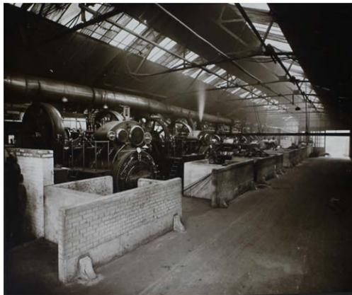
Inside the first Pelabon Workshop: the boiler room and steam engines
