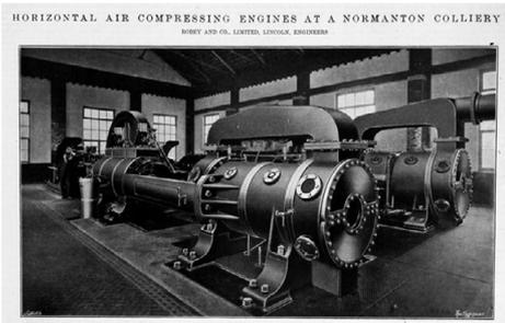
Horizontal air compressing engines at Normanton Colliery. Graces Guide, from The Engineer 01/06/1911
